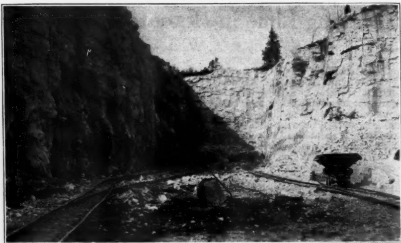
View of Quarry Breast Showing Drill Works.
